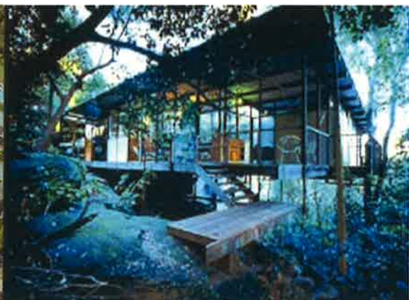
Figure 18: 80 The Bulwark (Source: Office of Environment and Heritage)
